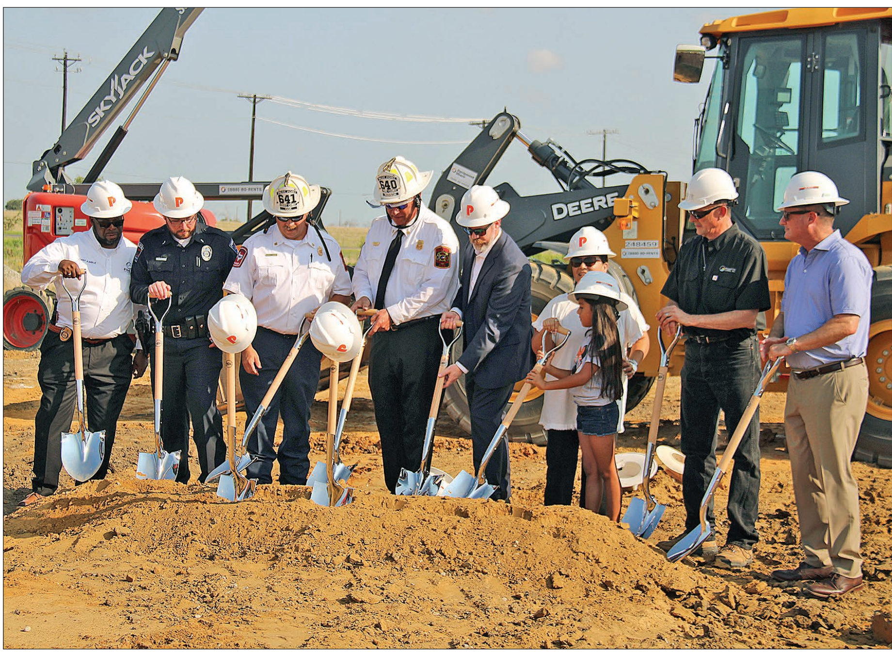
Pilot Point leaders and Mayor Elisa Beasley's daughter, Cara Beasley, joined by representatives from Plyler Construction and Brandstetter Carroll prepare to break the ceremonial dirt at Pilot Point's Station No. 2 groundbreaking on July 25. Abigail Allen/The Post-Signal
