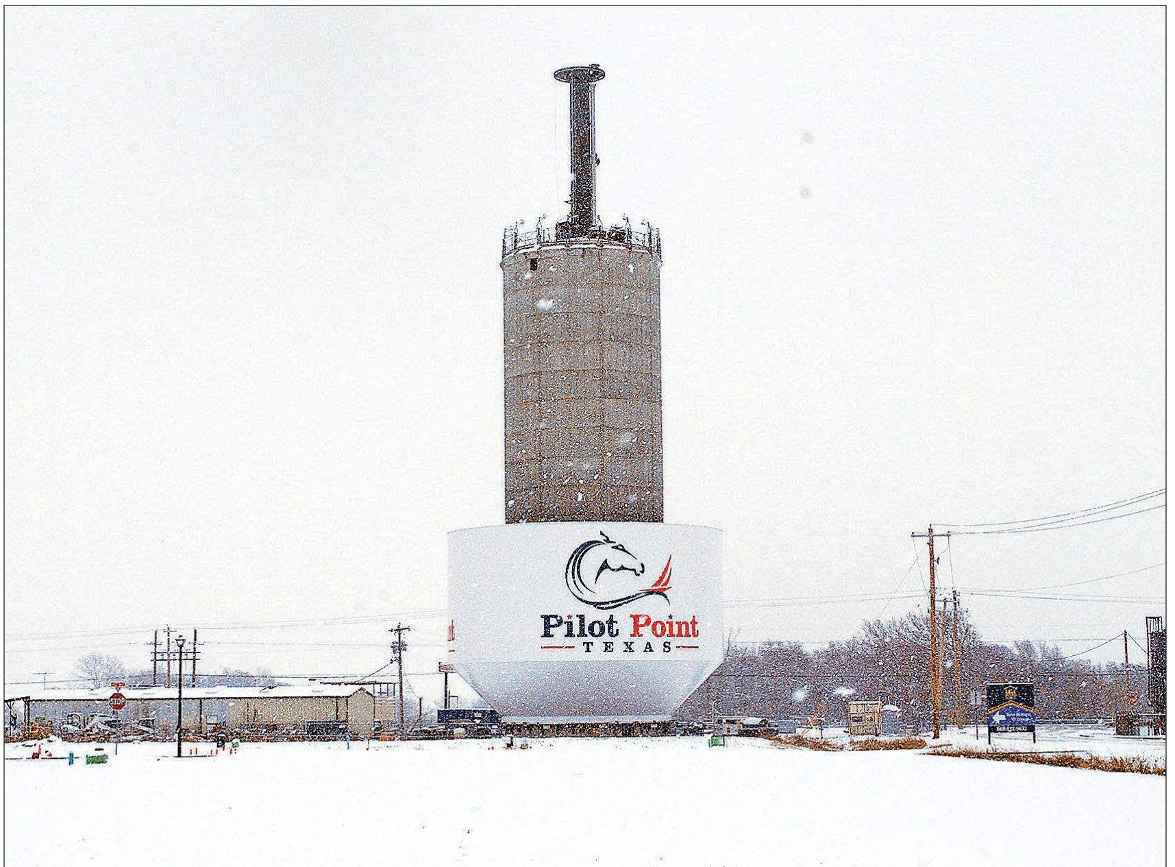
The bowl of Pilot Point's elevated storage tank rests during its final days on the ground before being raised on Tuesday.
