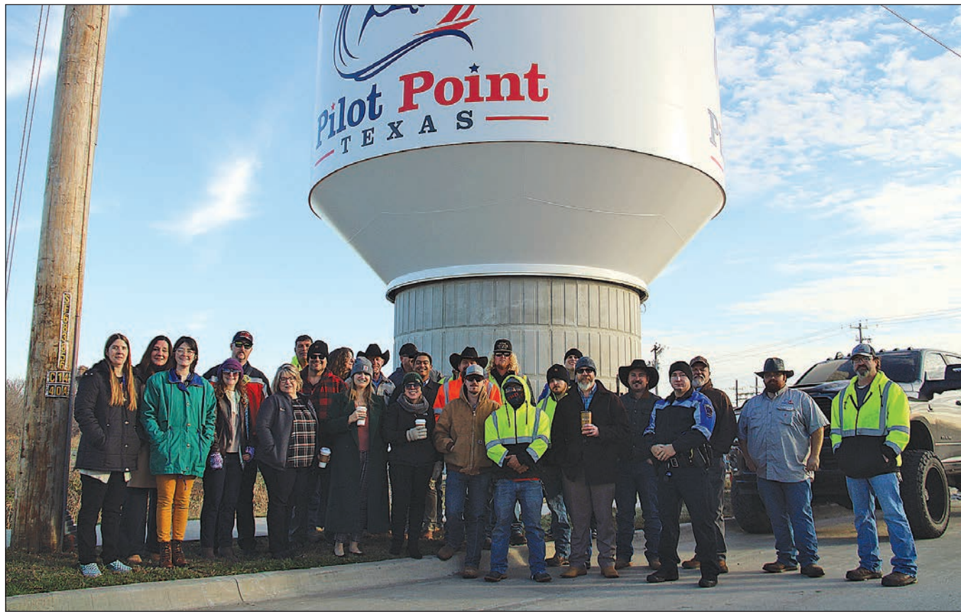
City staff poses for a photo in front of the rising bowl of Pilot Point’s new elevated water storage tank.
