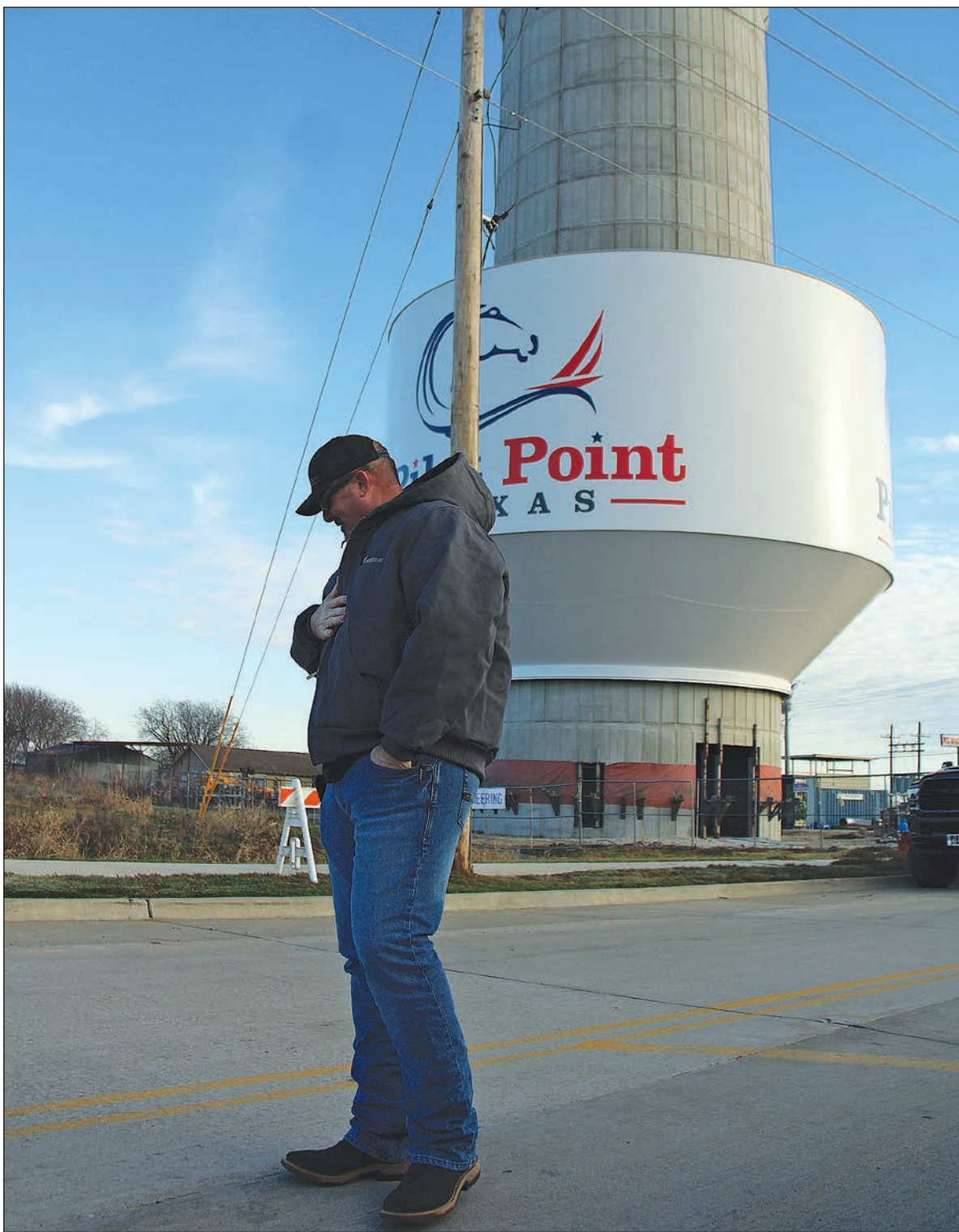
Former Pilot Point Public Works Director and current Wall Engineering employee Trent Vandagriff pauses before addressing the crowd as the city's new elevated storage tank rises in the background.
