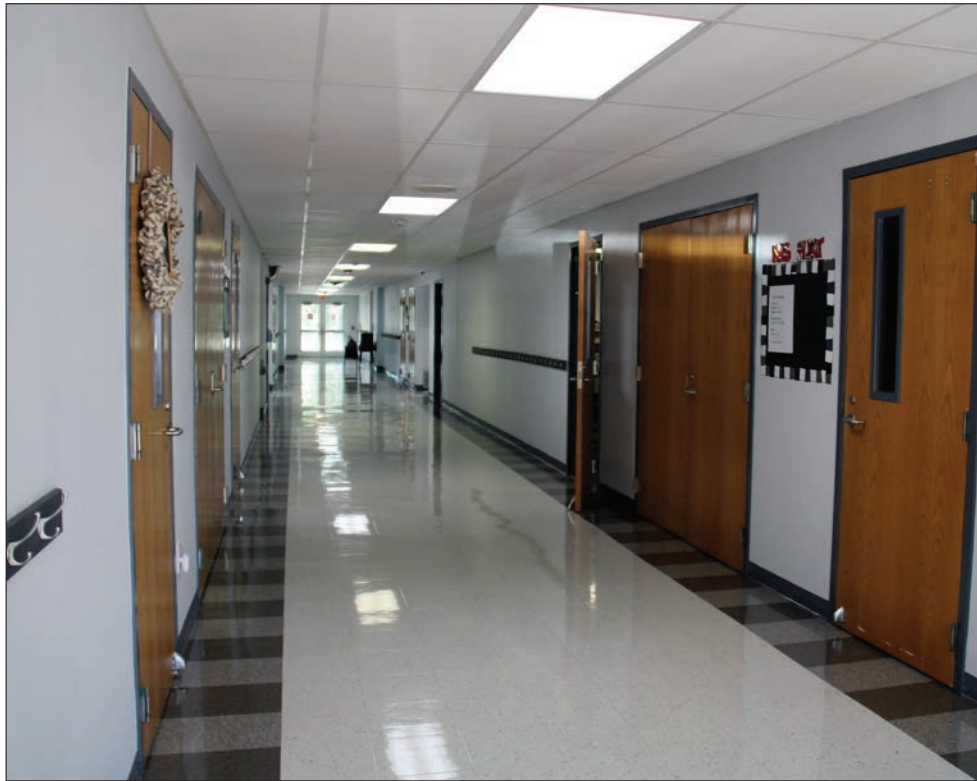
Volunteers and contractors have helped renovate a wing of the Tioga School, allowing the district to have additional room into which it can grow without needing to add more facilities yet.
